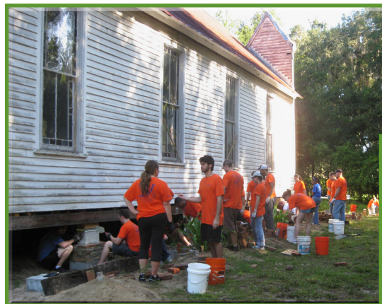
As a community service project, forty incoming UF law students became bricklayers for a day. They laid 120-year old bricks around new foundation piers supporting the historic Rochelle Church.
