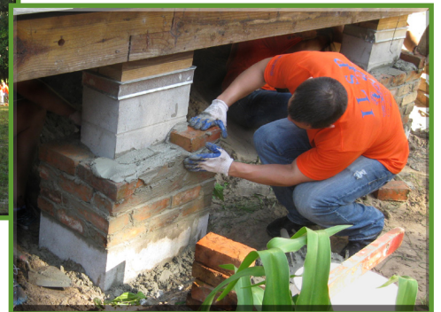
As a community service project, forty incoming UF law students became bricklayers for a day. They laid 120-year old bricks around new foundation piers supporting the historic Rochelle Church.
